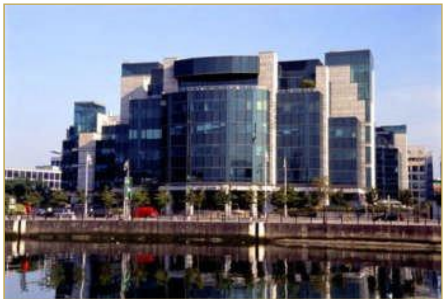
The newly built Financial Services Center in Dublin stands on the banks of the River Liffey. Ireland is bouncing back after the financial meltdown, which led to its bailout by the International Monetary Fund and the European Union in 2010.
