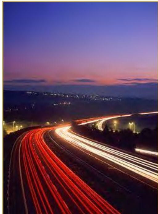
Expressway lit-up in the night, near Devon, England. The U.K. government's public spending in large infrastructure projects is intended to shield the economy from the adverse effects of the economic downturn to some extent.
